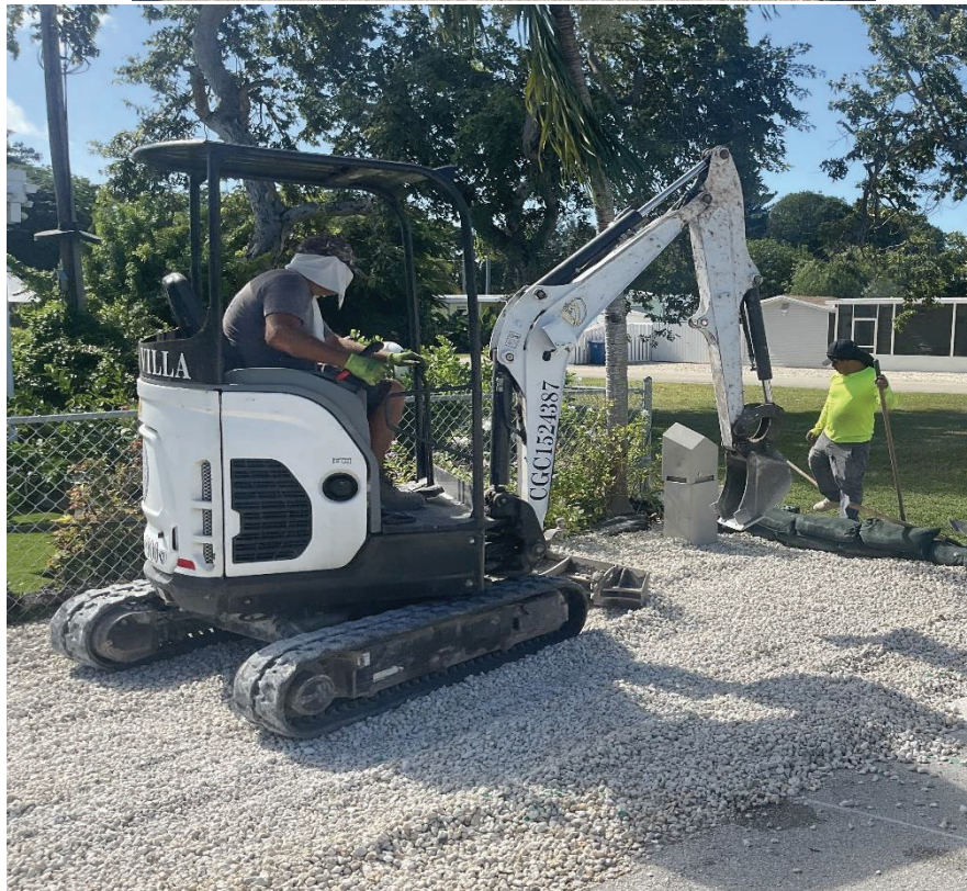
Figure 5 and 6. Installation of Conduit & Flovac Pedestal and Site Restoration for Collection System Monitoring Project.
