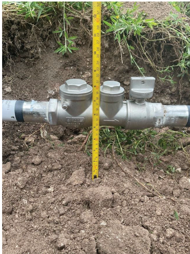
Figure 10 and 11. New SS Sewer Lateral Valve Assembly and Valve Box Installed.
