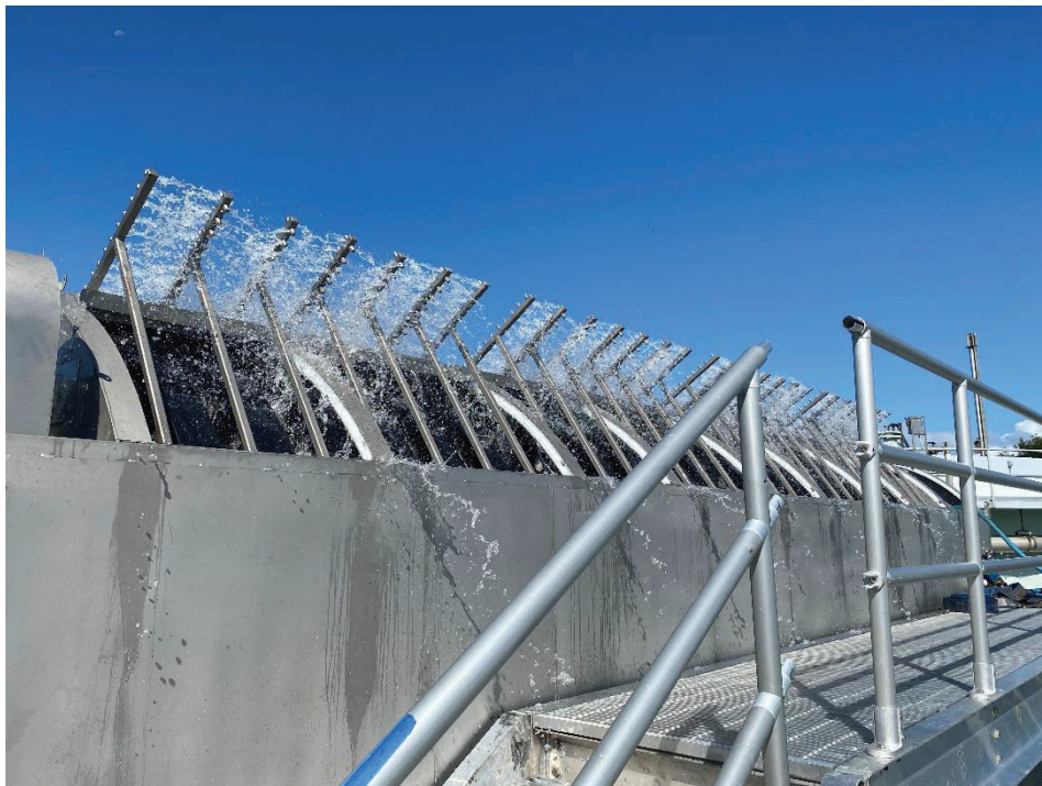
Figure 8. Spray Headers being tested during Start-up.
