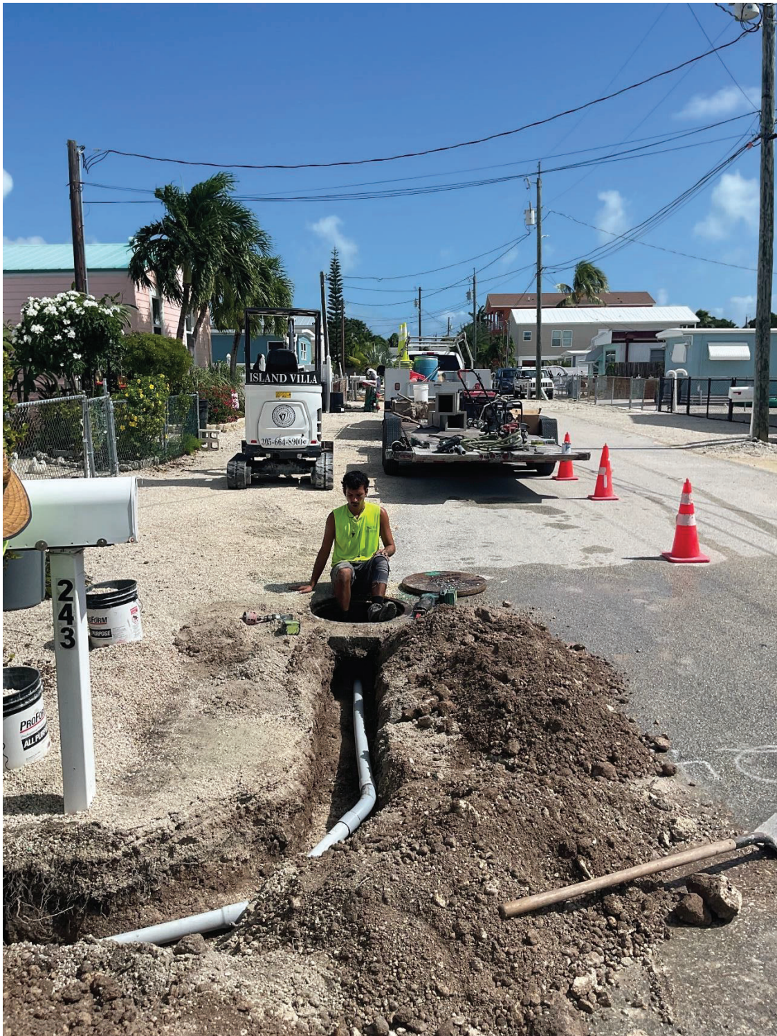
Figure 4. Install Conduit in Trench for Collection System Monitoring Project.
