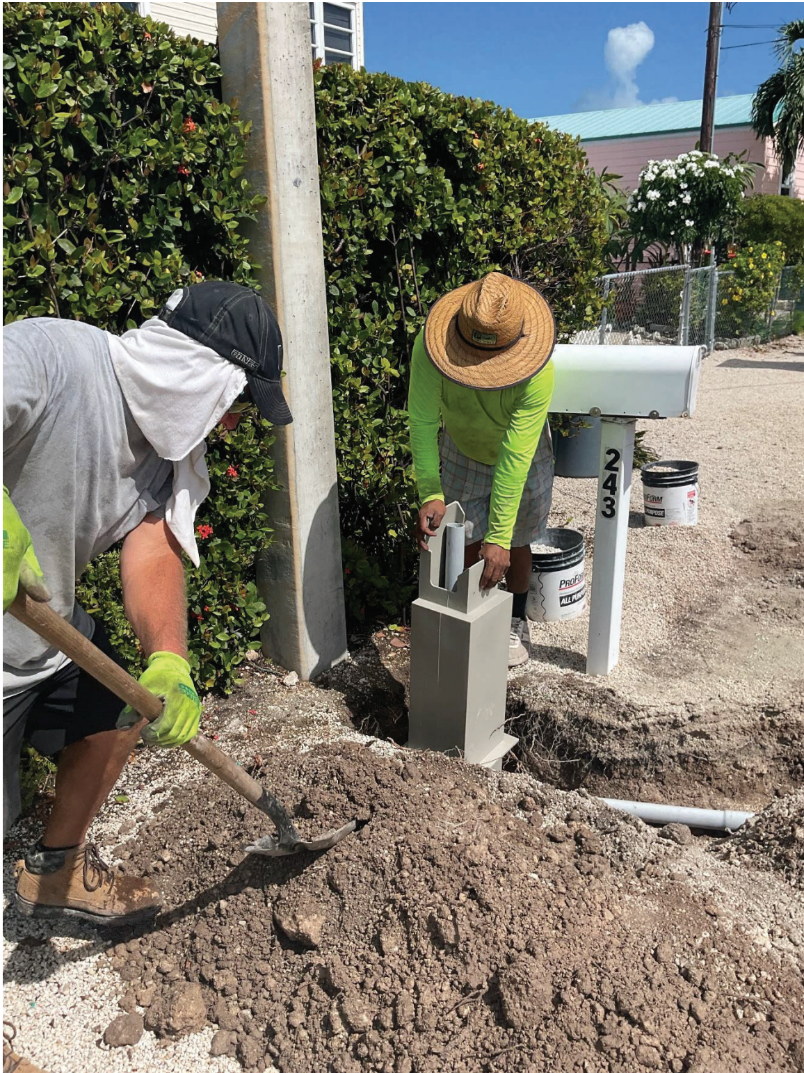
Figure 5. Install and Leveling of the Pedestal for Collection System Monitoring Project.
