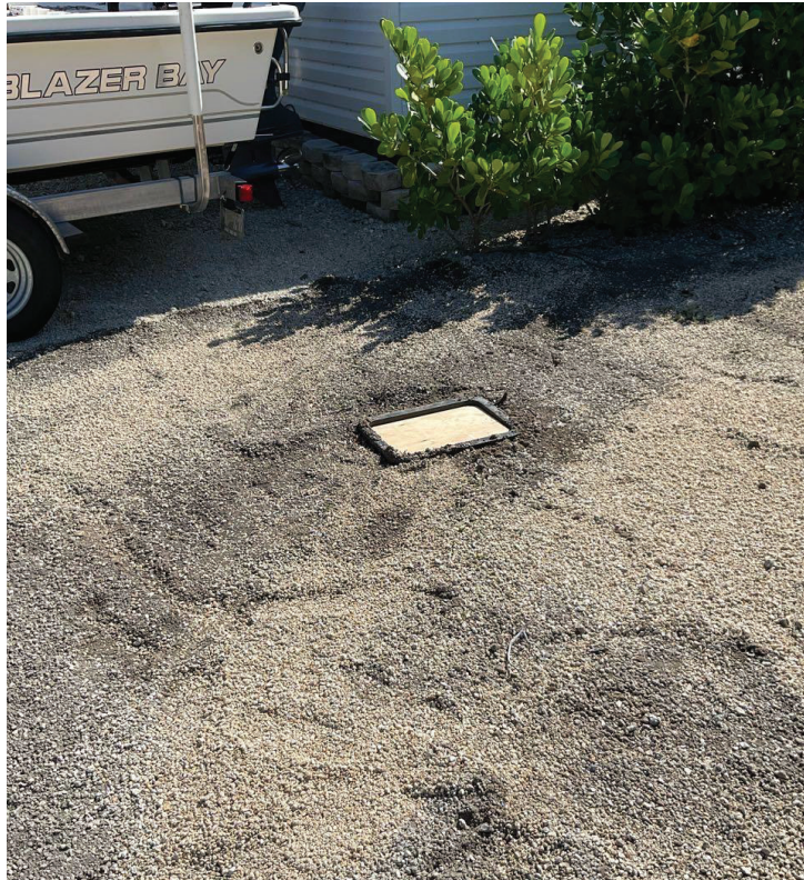
Figure 9 and 10. New SS Sewer Lateral Valve Assembly and Valve Box Installed.
