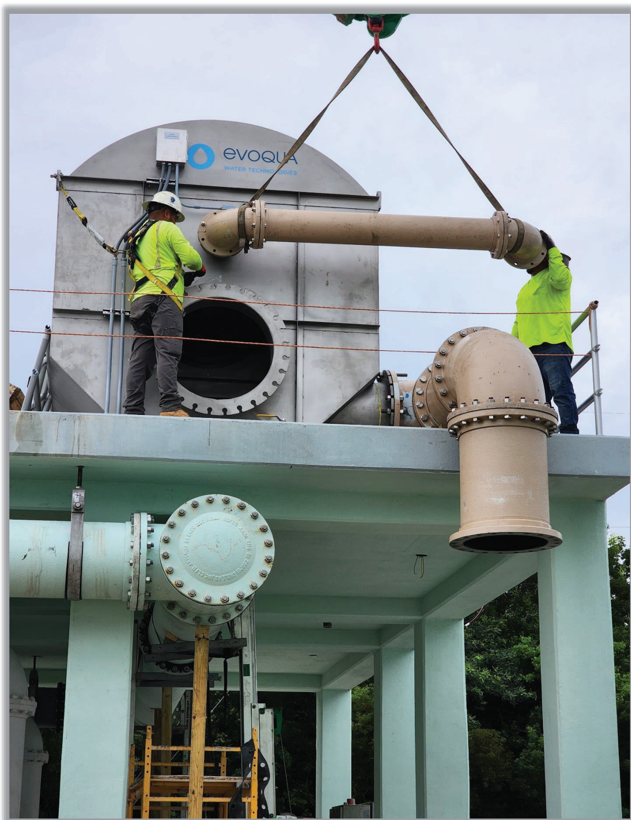
Figure7: Overflow and backwash piping installation
