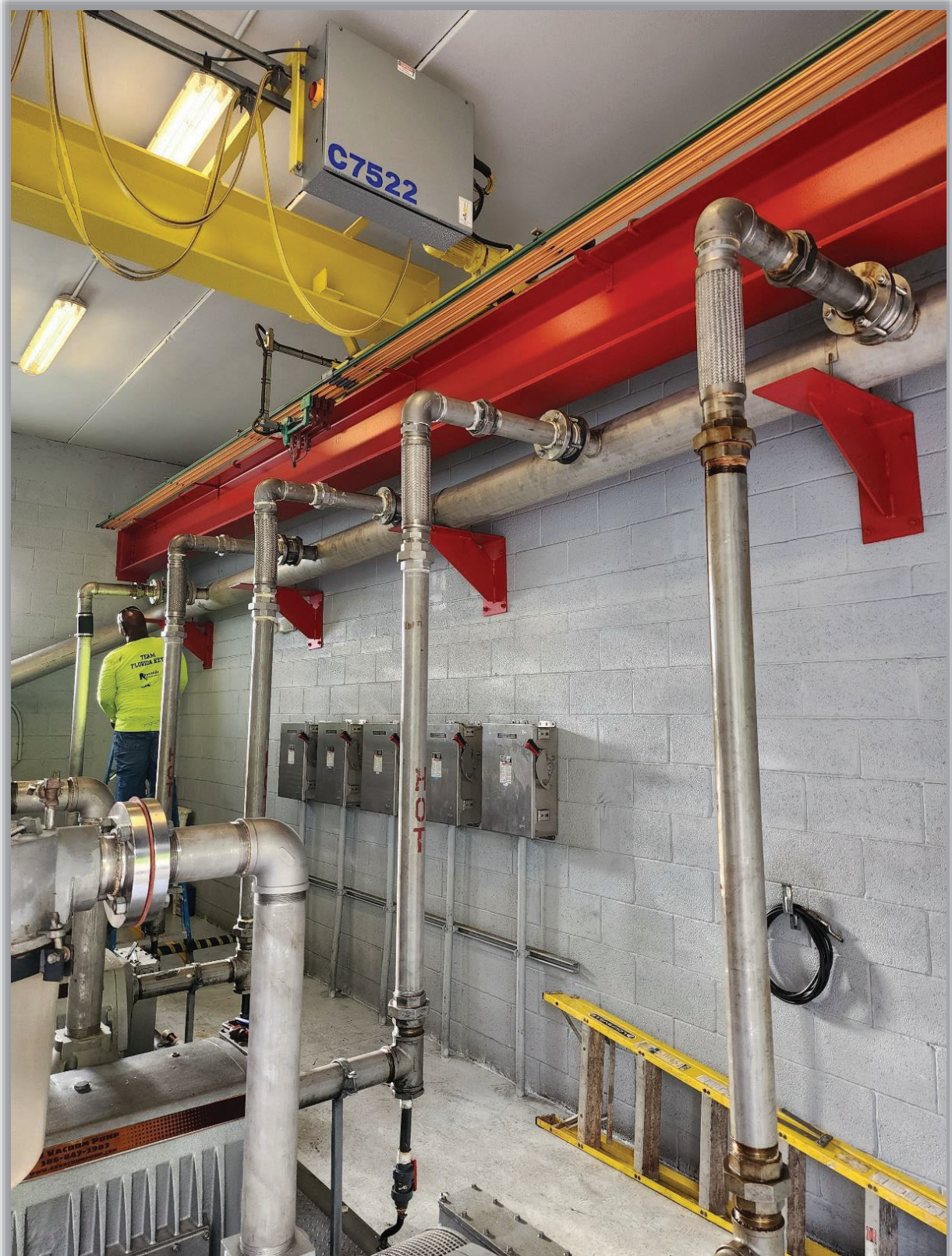
Figure 1: Odor control lines modified with new SS valves, 90 elbows, and flex piping at vacuum station JK
