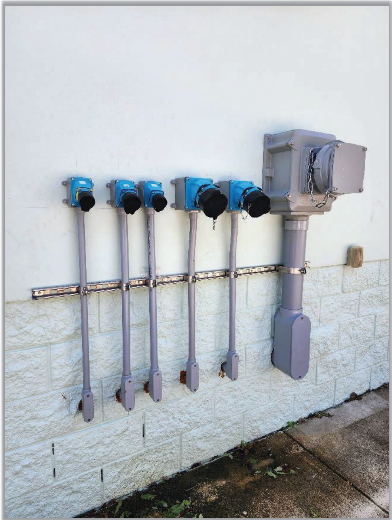
Figure 4: Wiring Terminated at All Outdoor Conduit Receptacles at Vacuum Station G
