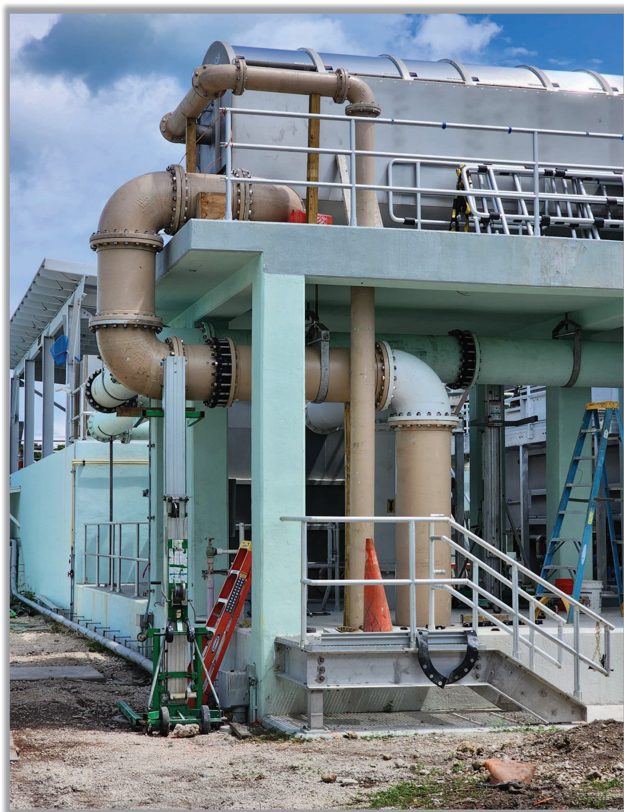
Figure 8: Overflow and backwash piping installation
