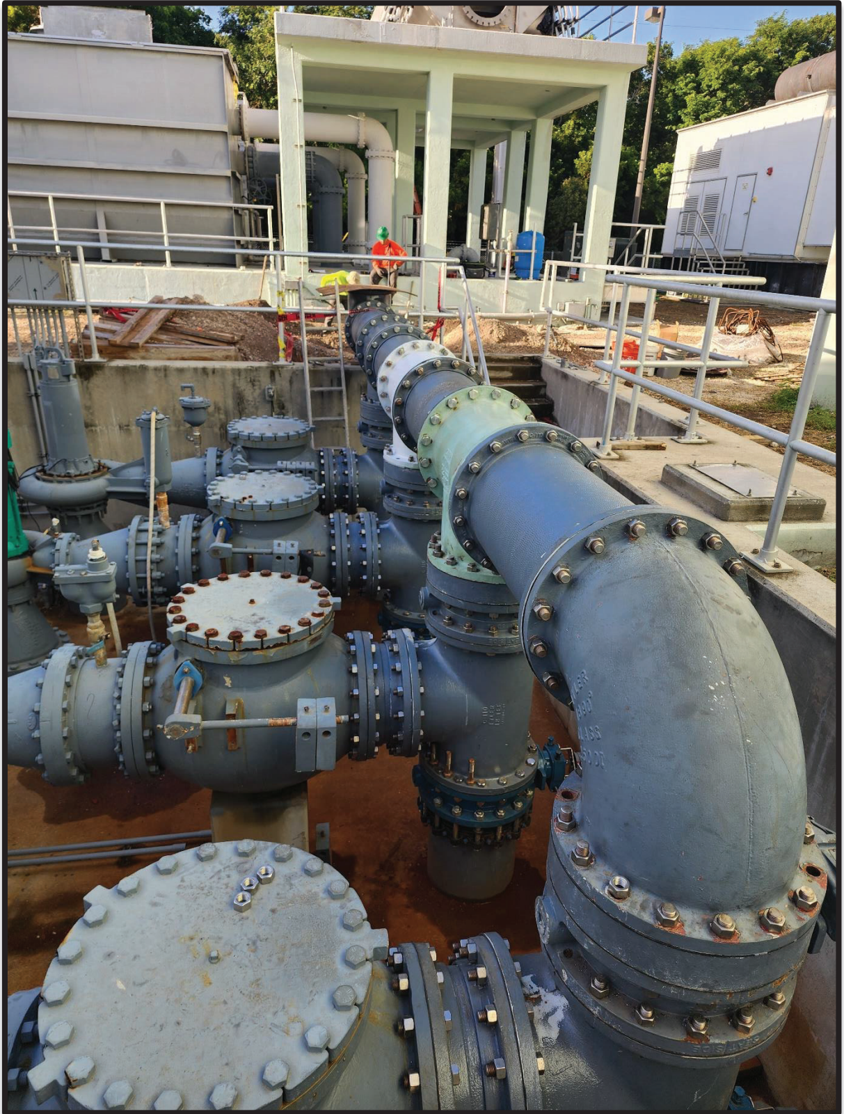
Figure 4: Newly Installed Booster Pump Piping
