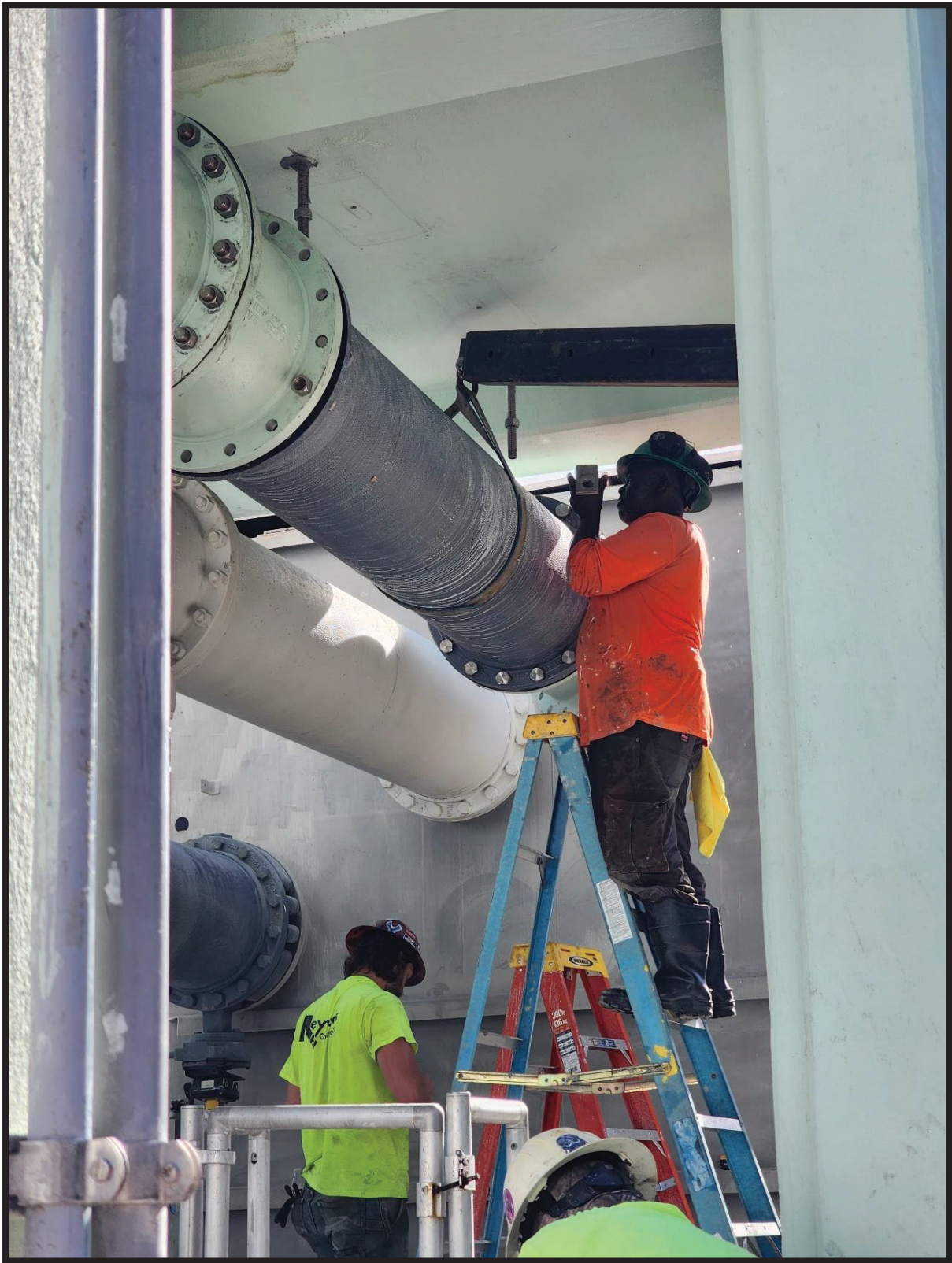
Figure 5: Boom Installed to Lull Forklift to Support 18" D.I. Spool Piece and 18" D.I. 45 Elbow During Installation of SS Pipe Hangers
