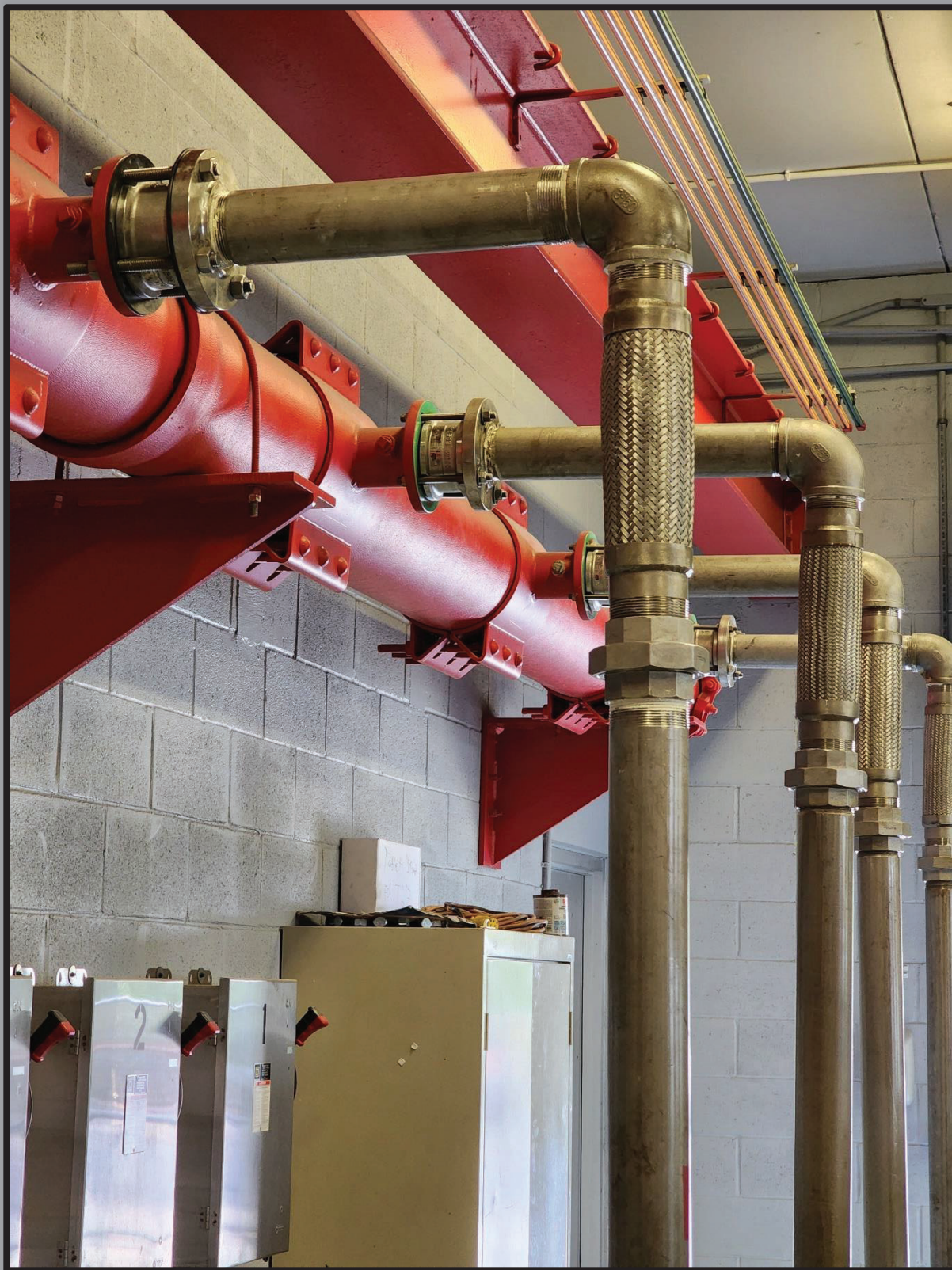
Figure 6: Replaced (4) 3" SS Odor Control Lines with New SS Tubing and SS Fittings at Vacuum Station A
