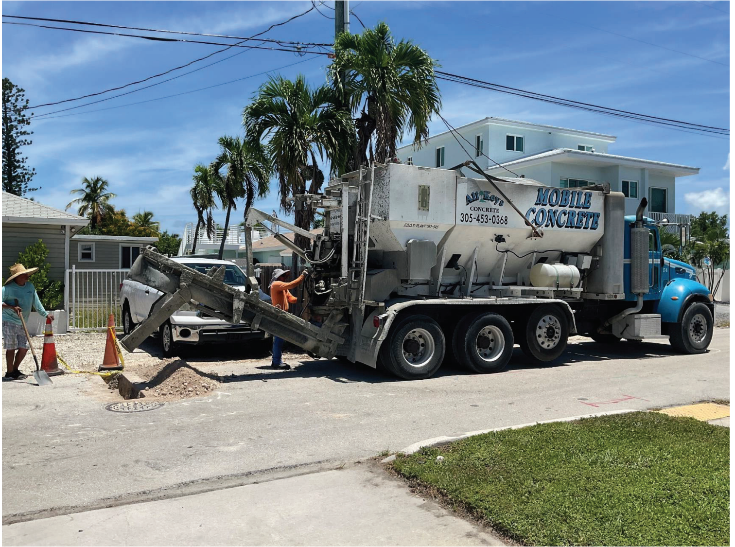
Figure 6: Flowable fill installation in Basin J/K
