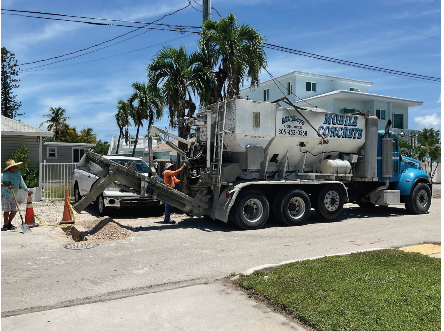
Figure 6: Flowable fill installation in Basin J/K
