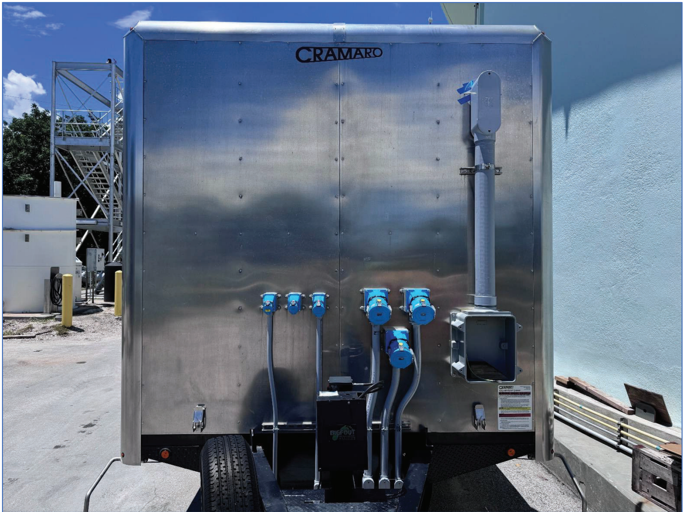
Figure 2: Emergency vacuum trailer front view. Power and control receptacles have been mounted and conduit has been installed.
