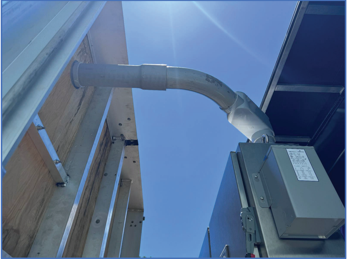
Figure 4: Overhead conduit
