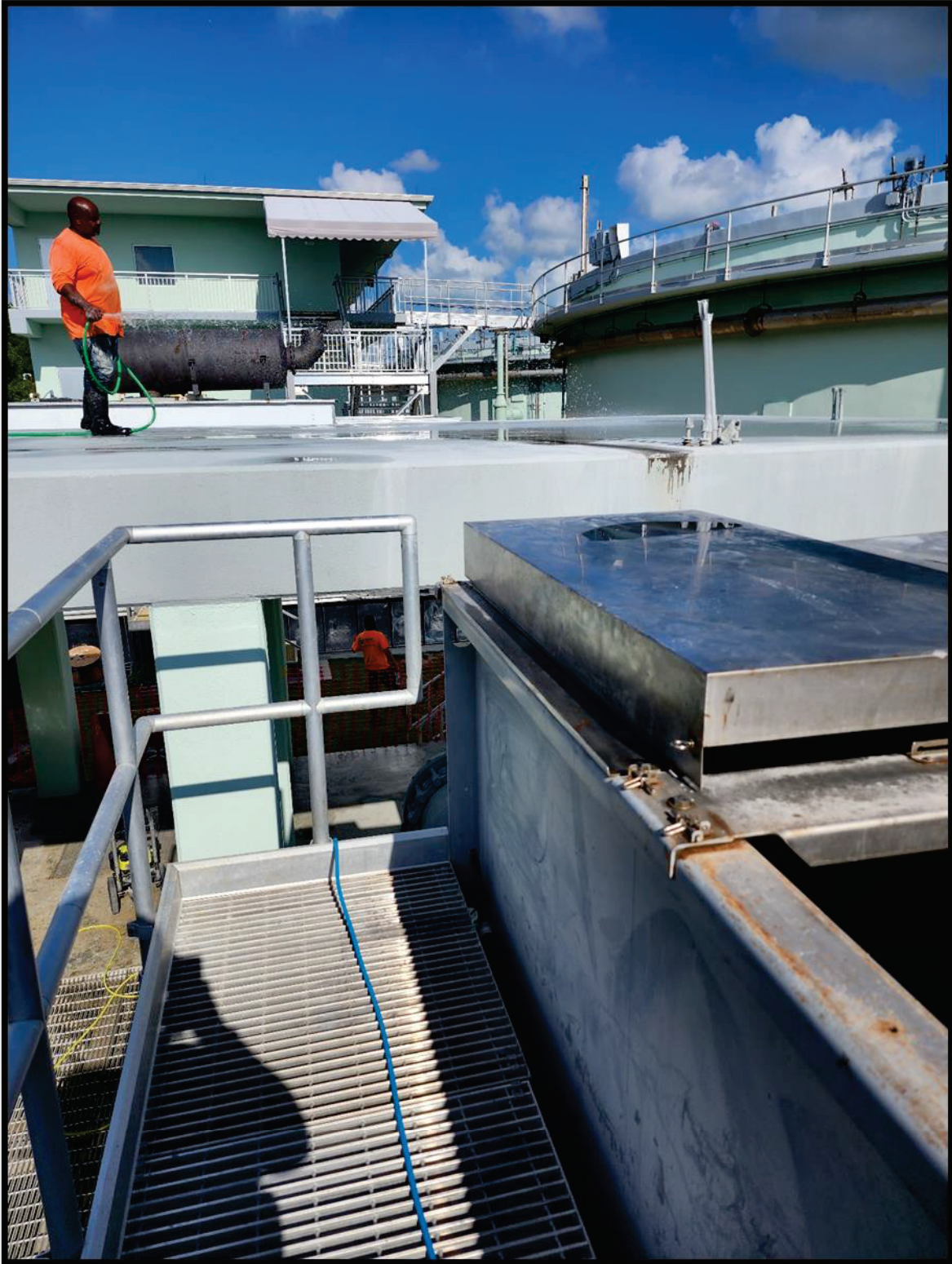
Figure 1: Reynolds Flooding Top of Concrete Disk Filters Platform at 9:20AM for Flow Test Observation
