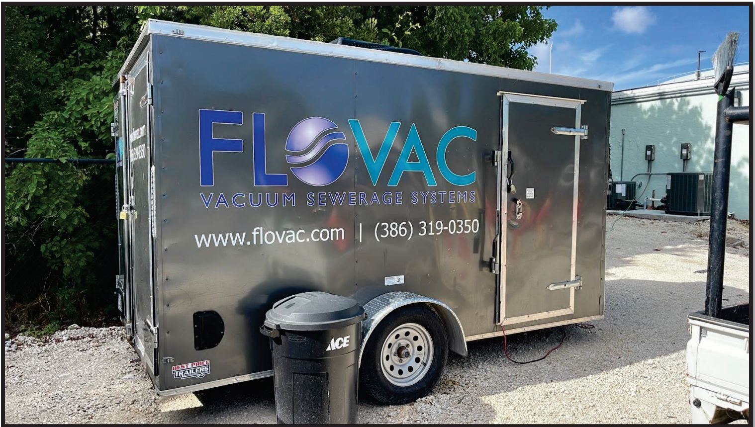
Figure 6: Flovac Valve Rebuild Trailer on Site at the WWTP for KLWTD Vacuum Monitoring
