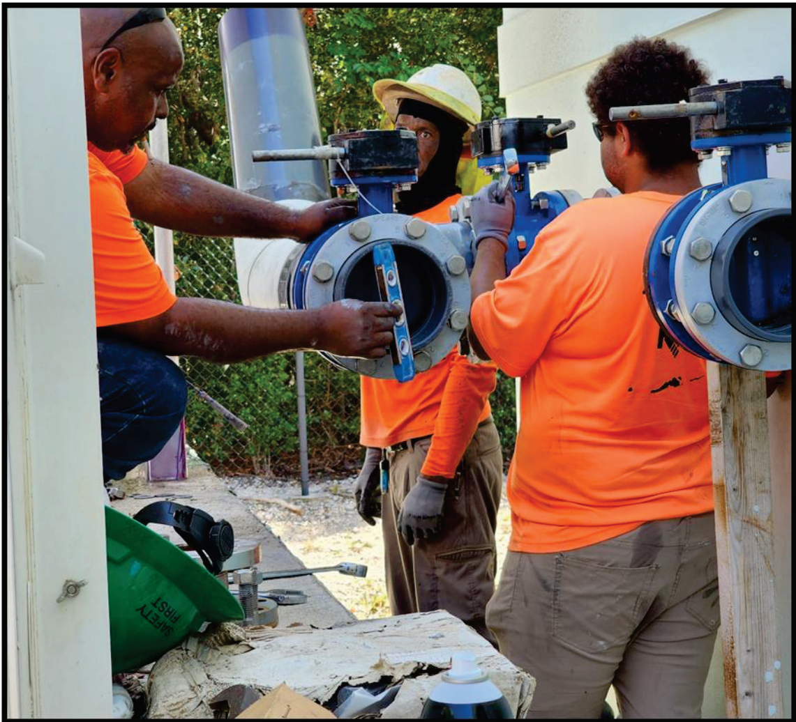
Figure 4: Installing new 8" Butterfly valve, 8"x8" PVC TEE, 8"x6" Reducer, and 6" Plug Valve to Odor Control Piping at Vacuum Station JK
