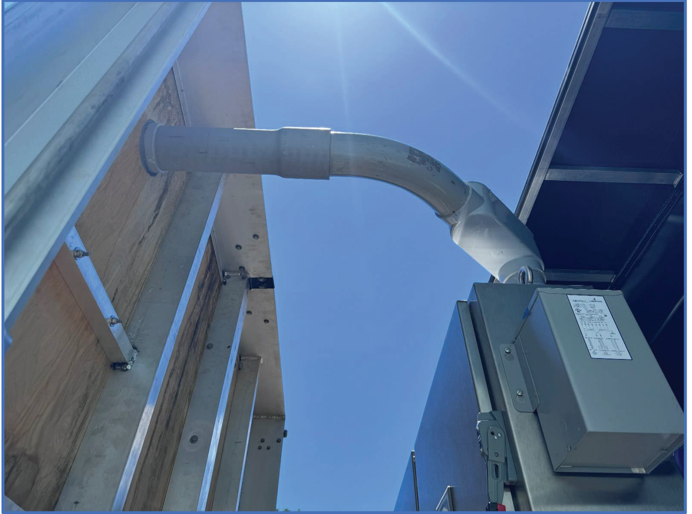
Figure 4: Overhead conduit
