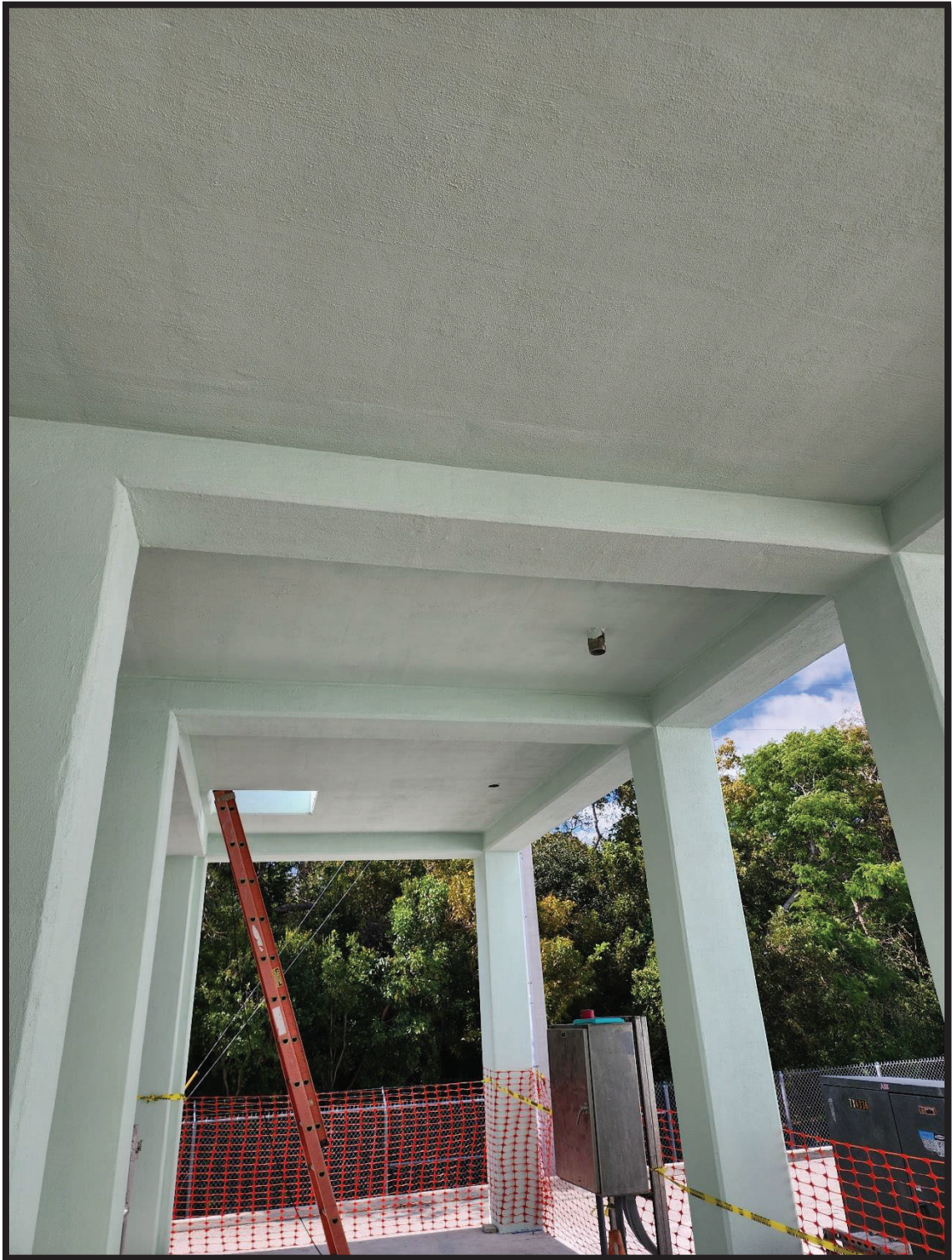
Figure 3: Filter Platform Bottom View
