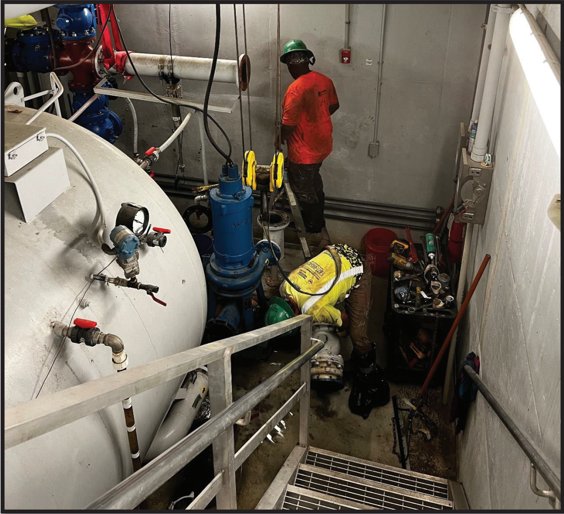
Figure 4: Shutdown at G on April 4, 2024. Reynolds removing effluent valve manifold.
