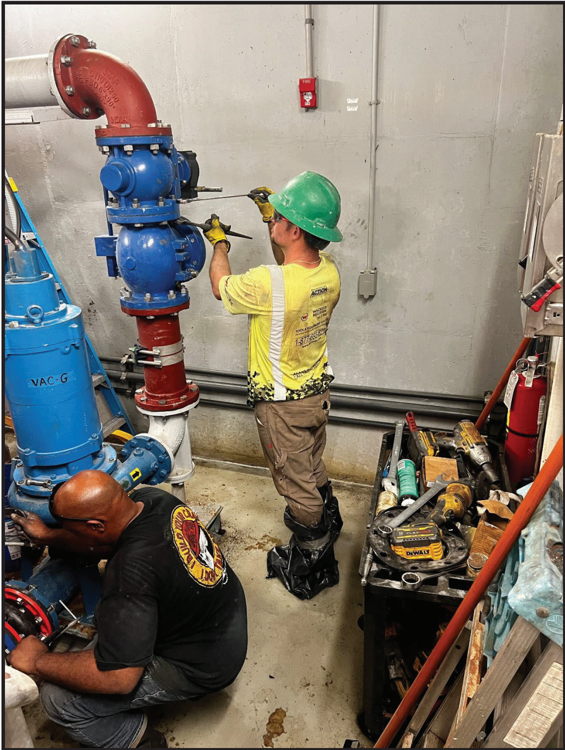
Figure 4: Shutdown at G on April 4, 2024. Reynolds installing new effluent valve manifold.
