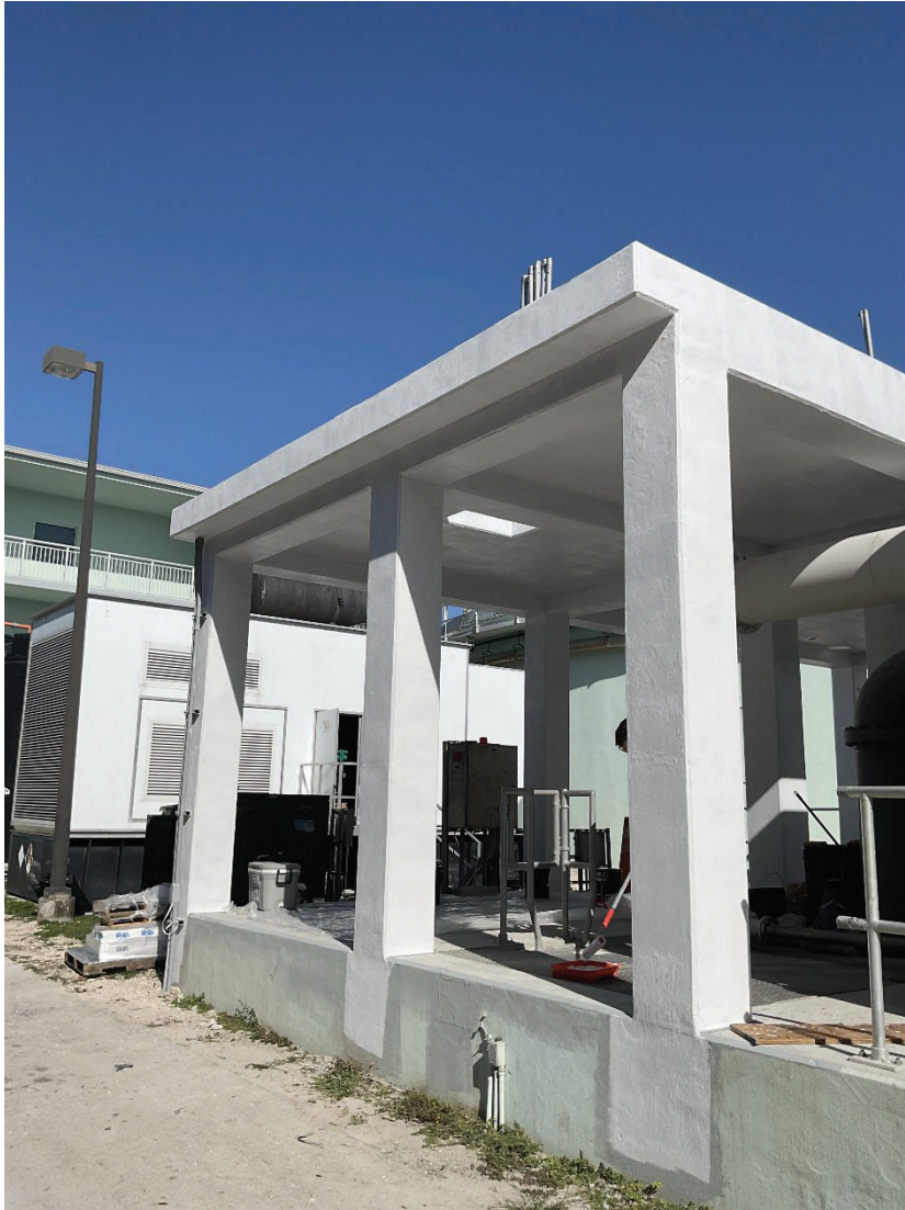
Effluent Filtration Upgrades Project: Front of elevated platform
