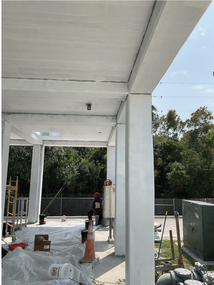
Effluent Filtration Upgrades Project: Coat 2 of 3 on the elevated platform
