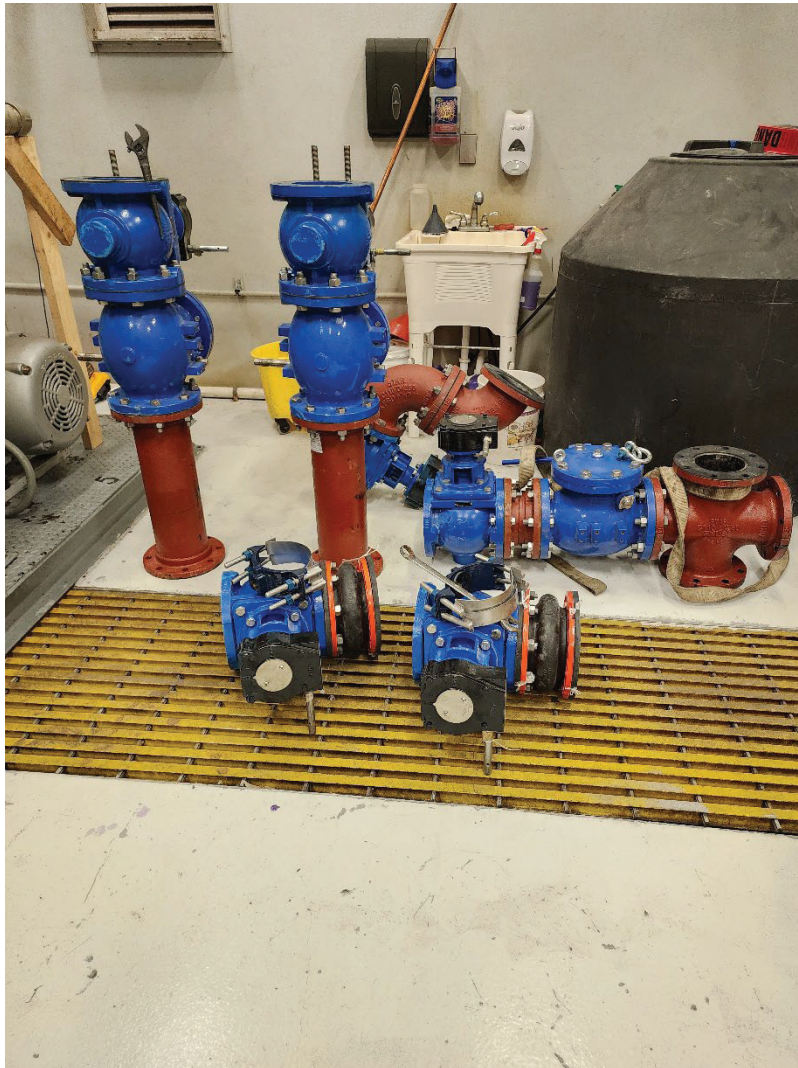
Vacuum Stations Modifications Project: Effluent valves and manifolds assembled and prepared for installation as part of the March 21, 2024 shutdown at Vacuum Station D
