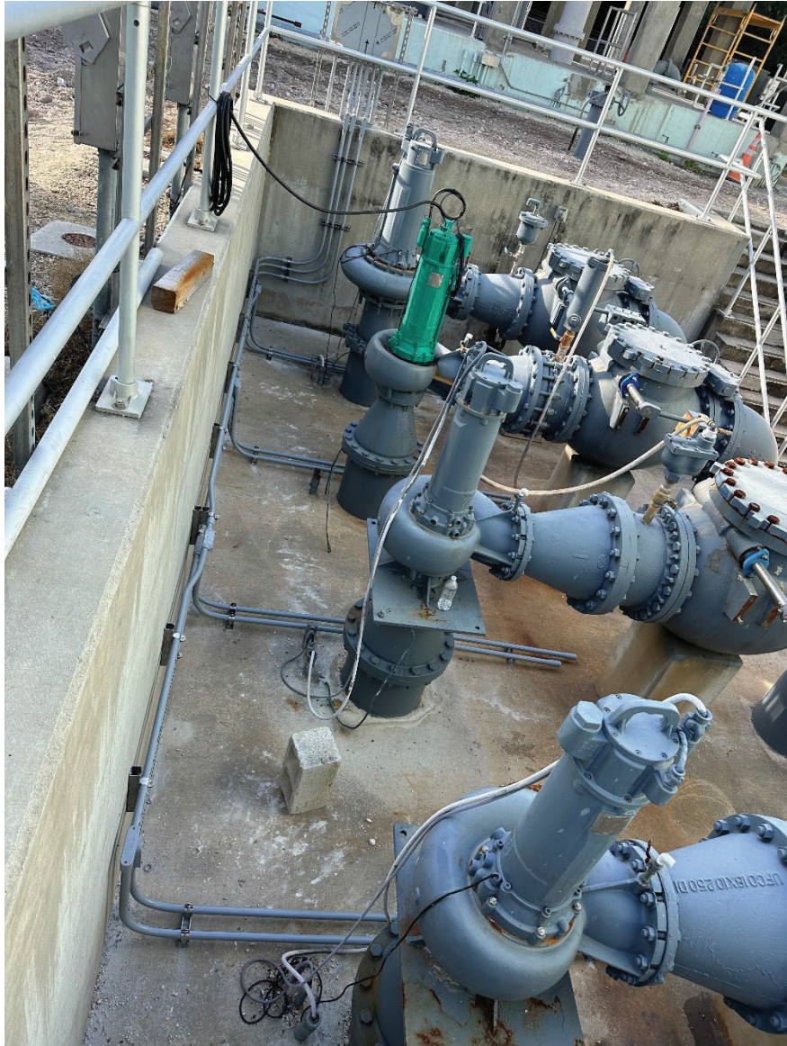
Effluent Filtration Upgrades Project: New electrical conduit servicing the booster pumps
