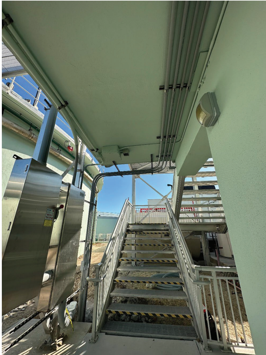
Effluent Filtration Upgrades Project: New electrical conduit servicing new filter
