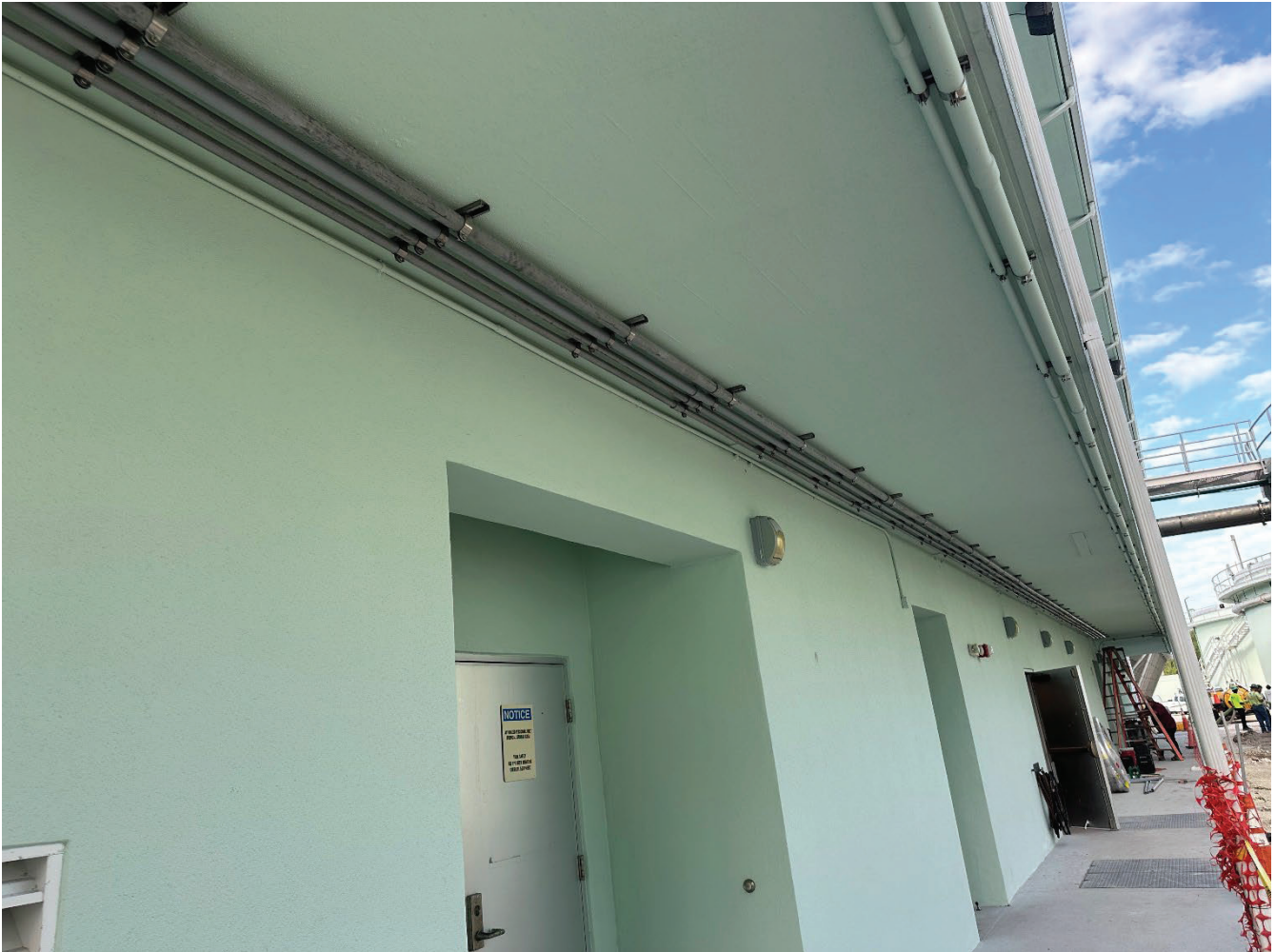
Effluent Filtration Upgrades Project: New electrical conduit servicing new filter
