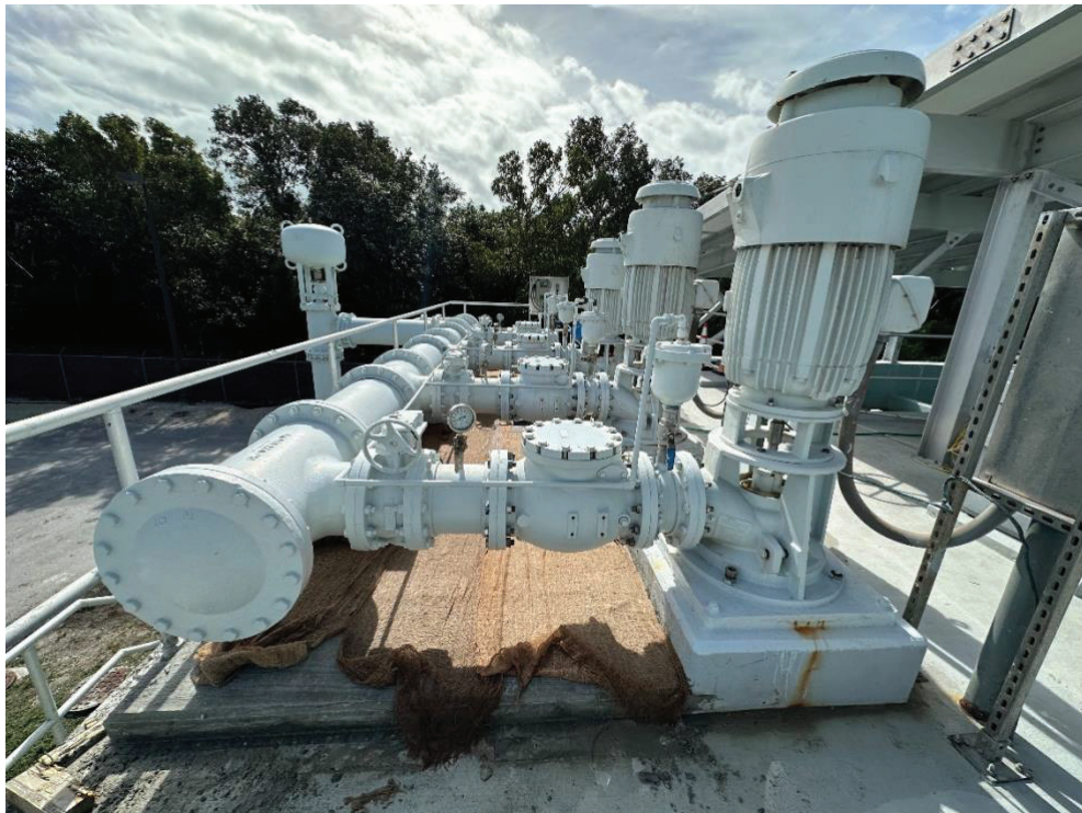
Effluent Filtration Upgrades Project: Pump slab after removal of forms
