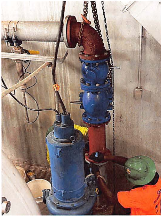
Vacuum Stations Modifications: West (left) and East (right) pump discharge valves installed at Vac Station I
