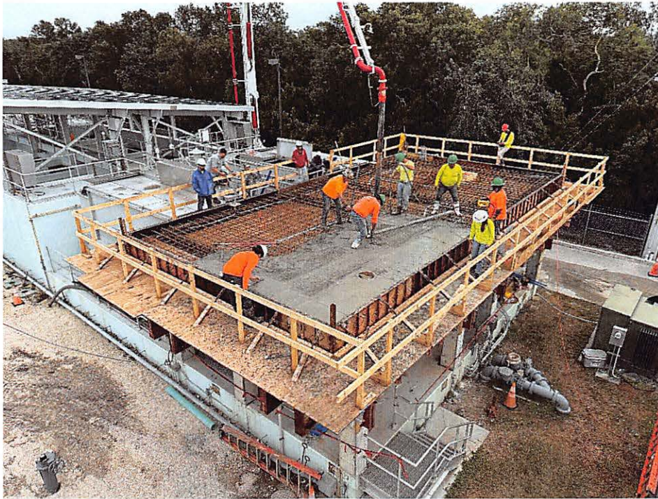
Effluent Filtration Upgrades Project: Concrete pour, top of filter platform
