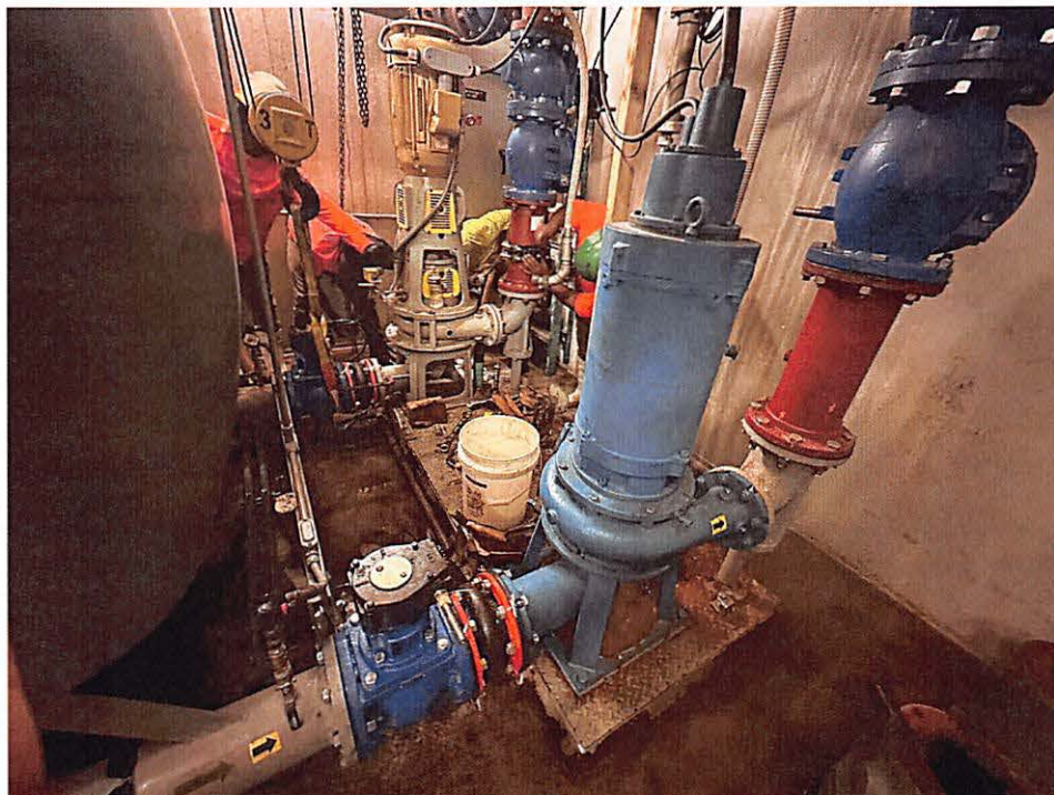
Vacuum Stations Modifications: All valves installed at Vac Station I
