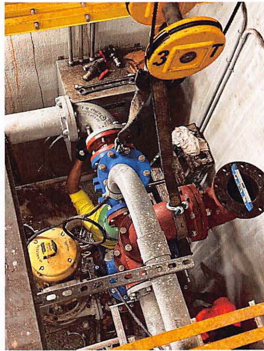
Vacuum Stations Modifications: West (left) and East (right) pump discharge valves installed at Vac Station I
