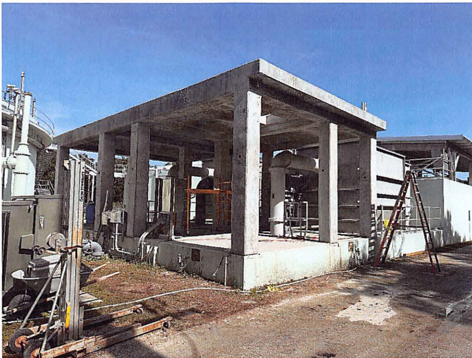
Effluent Filtration Upgrades Project: Filter platform after removal of forms
