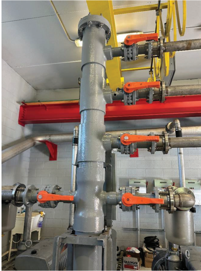
Vacuum Stations Modifications: New vacuum pump pipe tree installed at Vac Station J/K
