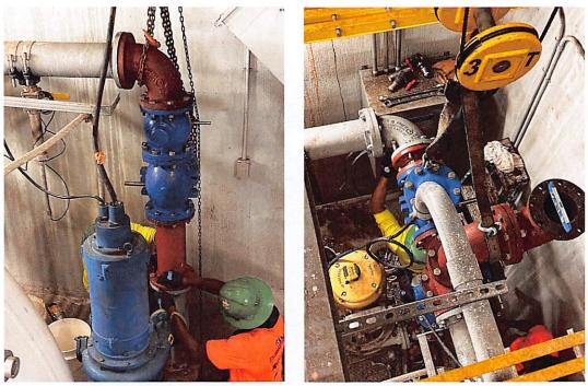
Vacuum Stations Modifications: West (left) and East (right) pump discharge valves installed at Vac Station I
