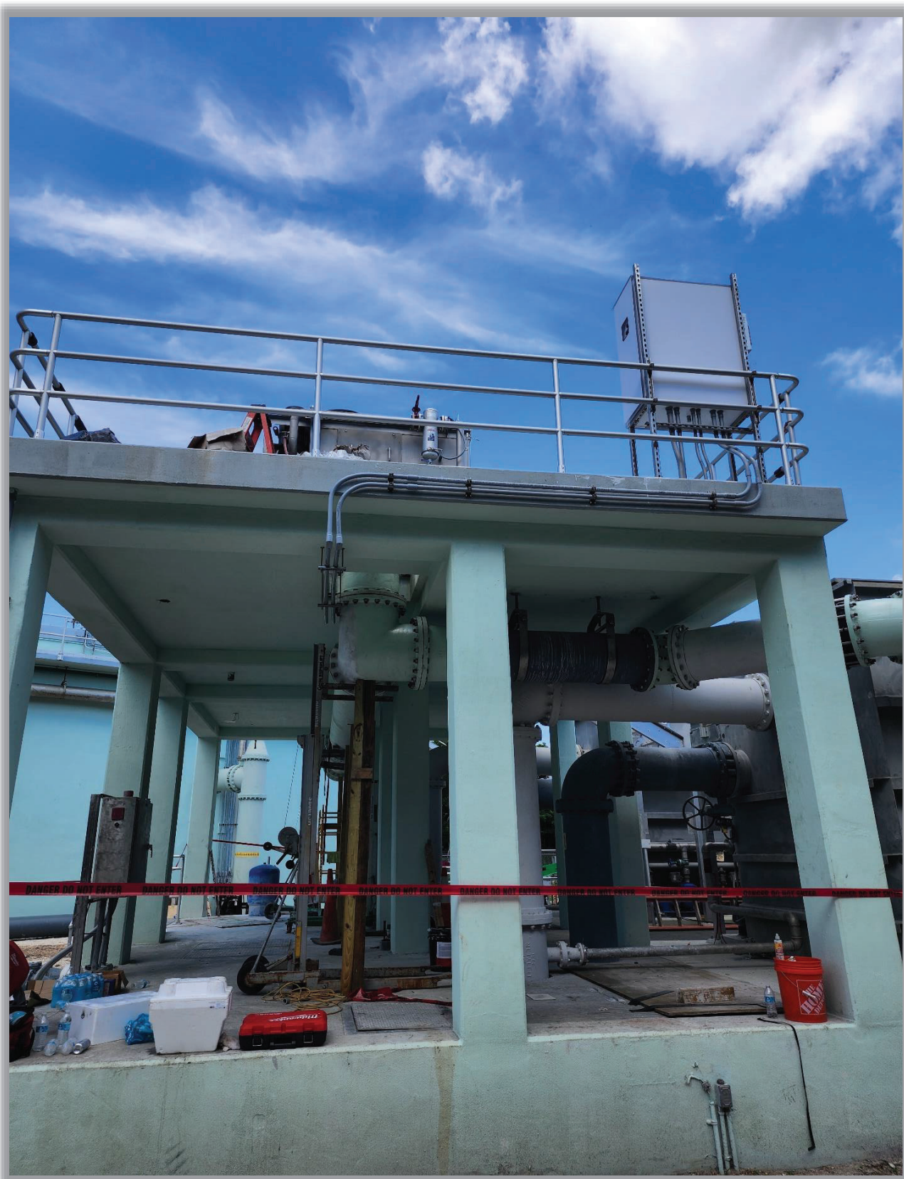
Figure 11: Installing conduits for the disk filter control panel
