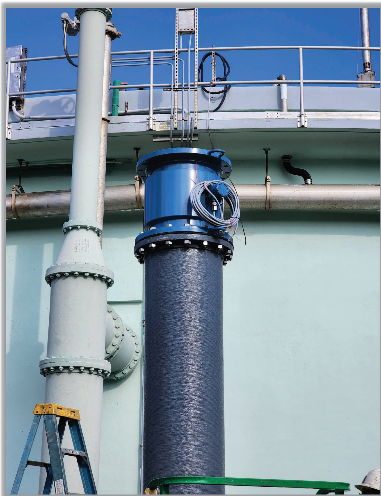
Figure 9: Installed new flow meter on influent disk filter pipeline
