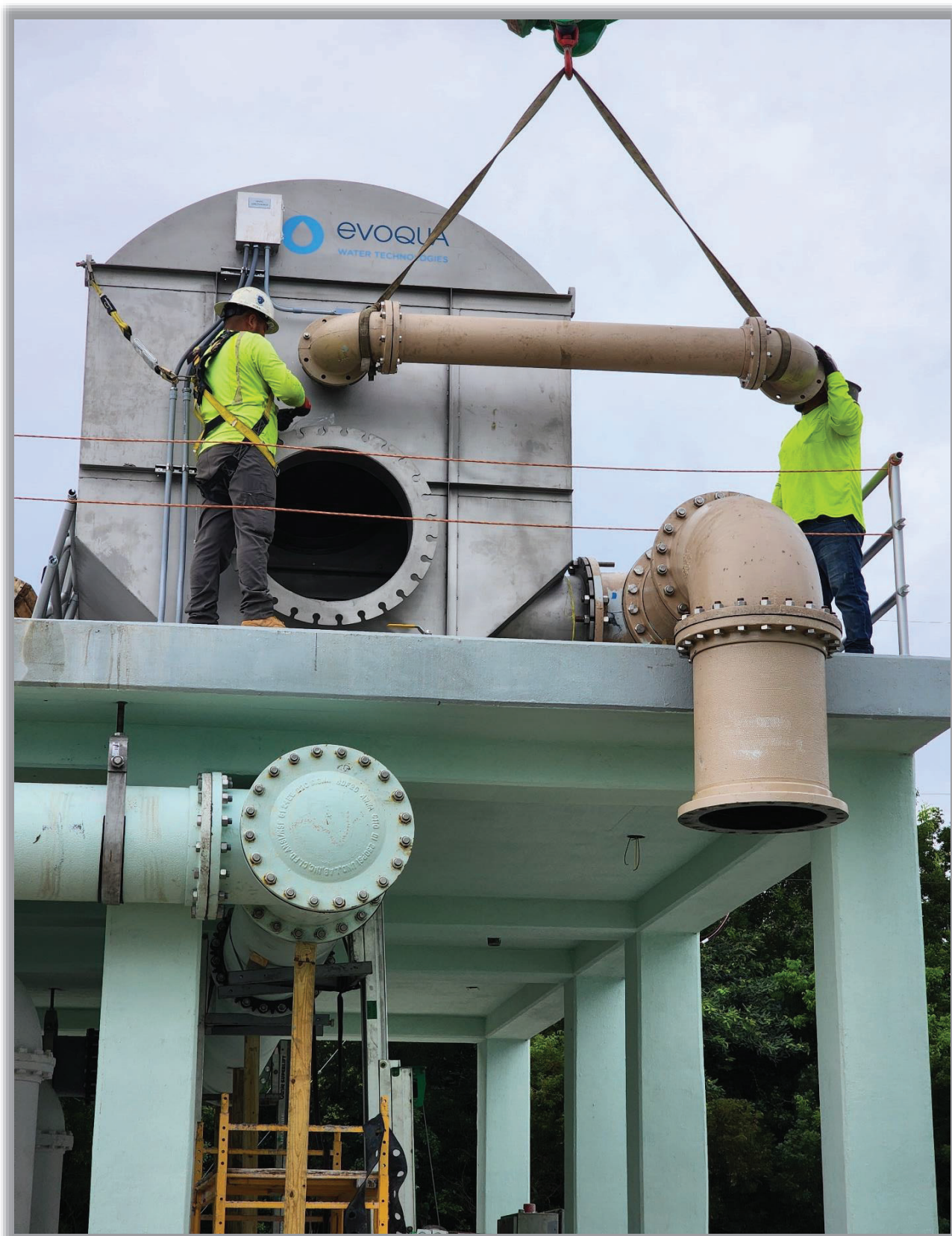
Figure7: Overflow and backwash piping installation
