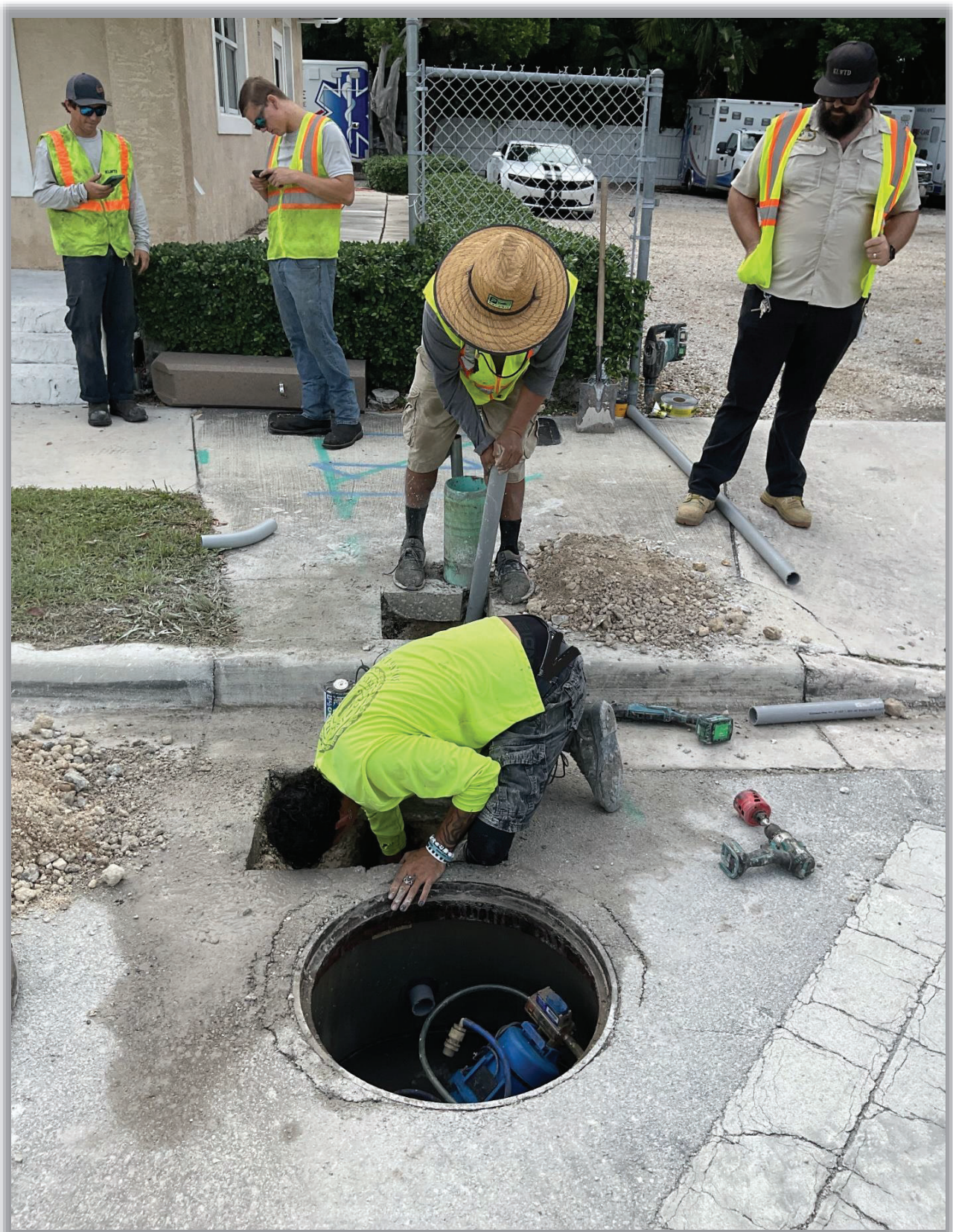
Figure 6: IVC installing conduit for Flovac Monitoring System in JK
