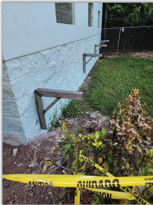
Figure 2 and 3: Pipe Supports for Force Main Connection and Bollards Installed at Vac Stations
