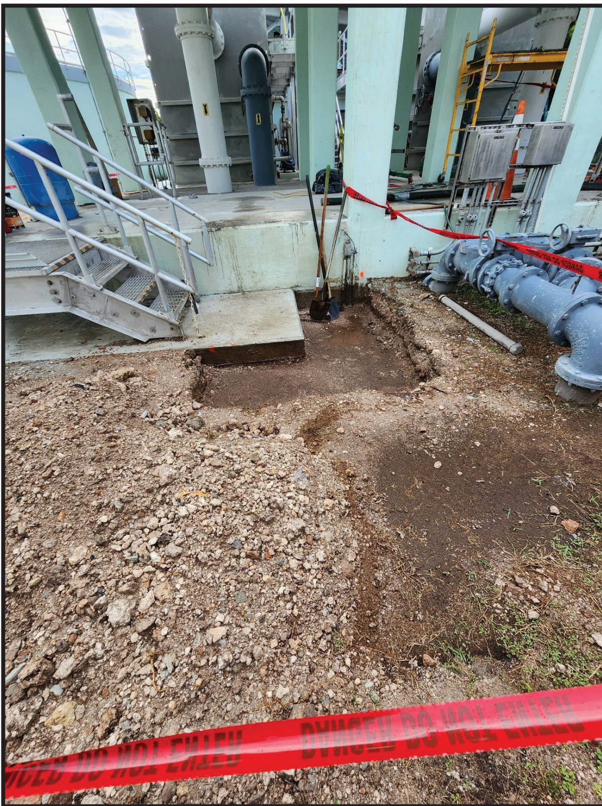
Figure 3: Trench to Extend Concrete Pad for Stair Leading Up to Existing Filters
