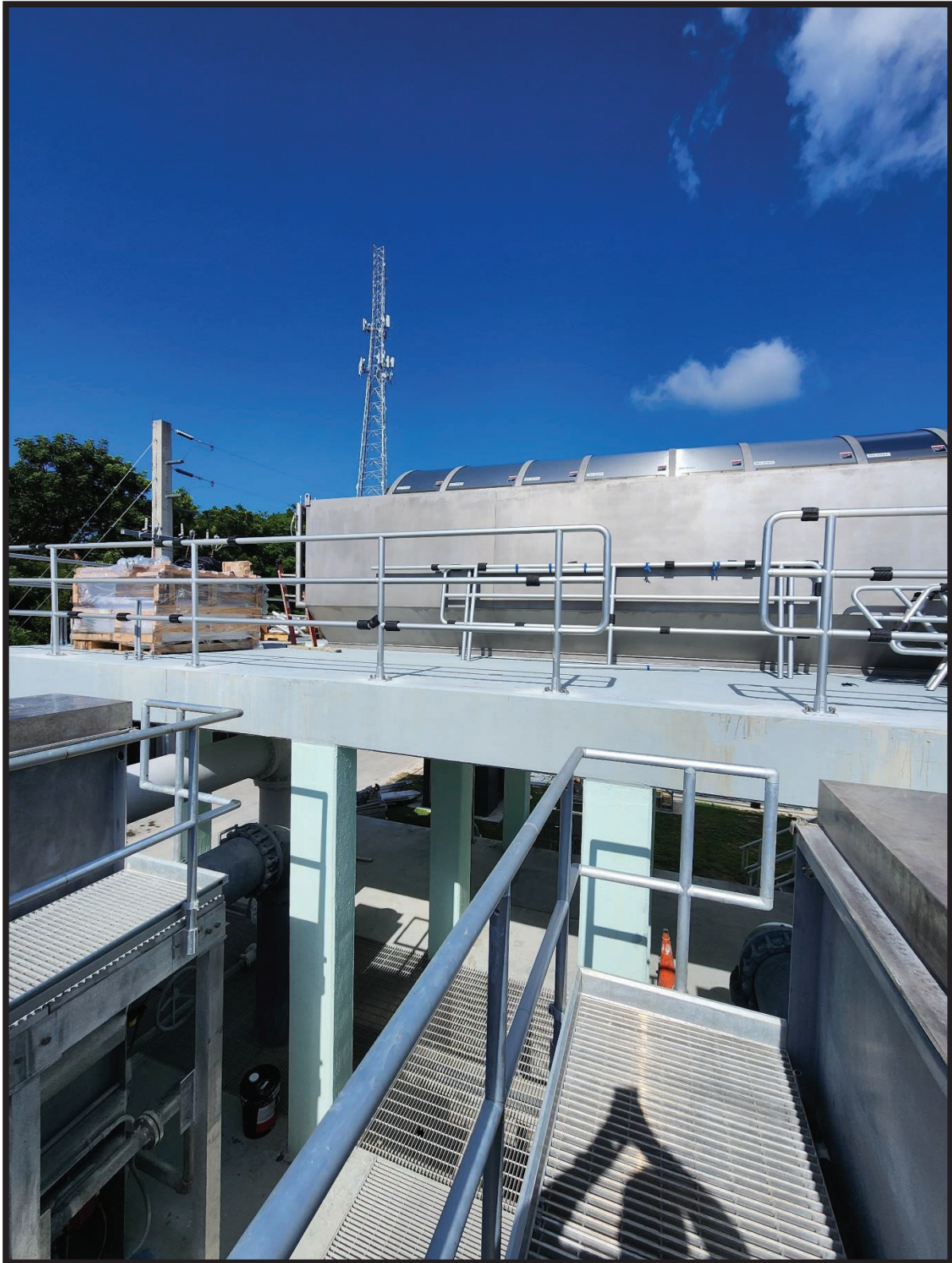
Figure 1: New Disk Filter Has Been Placed at Top of Concrete Platform and Handrails have been installed on South and East sides of deck
