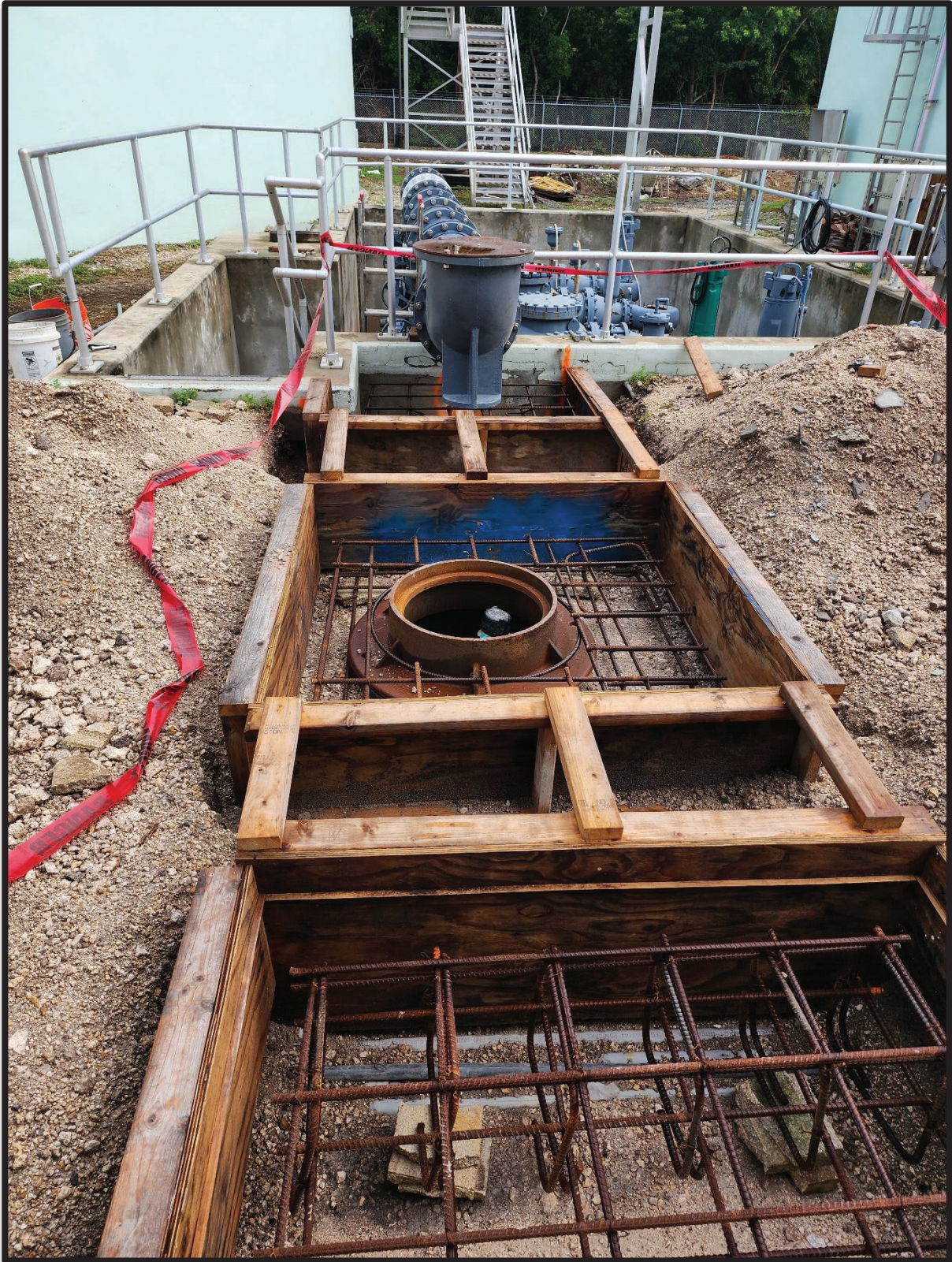
Figure 2: Concrete Forms Installed with Structural Rebar Between Disk Filter Platform and Booster Pumps Basin
