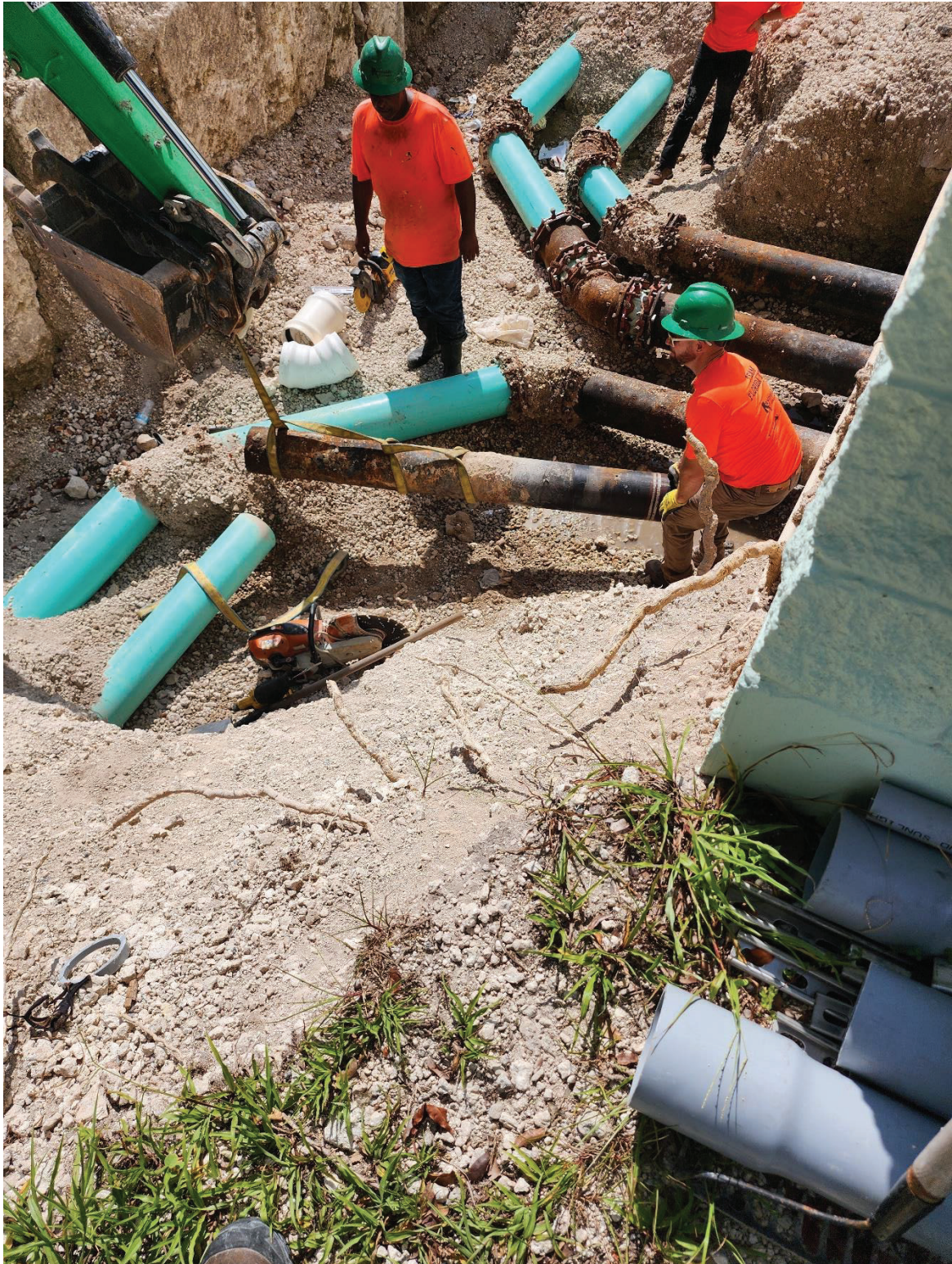
Figure 4: Installing New 8"SDR-21 PVC with 2 New 8"SDR-21 PVC 45 Bends at North Exterior of Vacuum Station A
