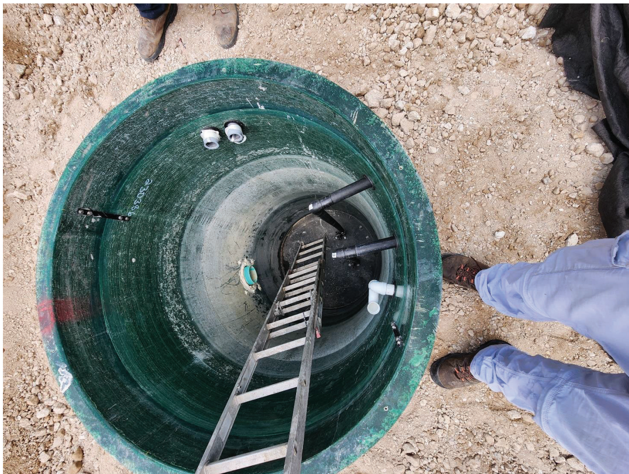
Figure 5: New Bases Installed to Interior of New Lift Station Well at Keys Holdings Lift Station
