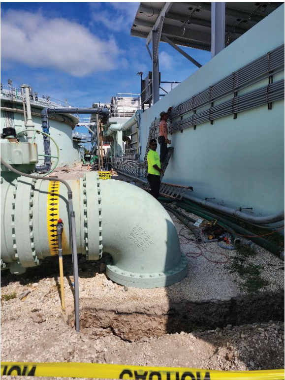
Figure 10 and 11. Conduit run along the side of the chlorine contact chamber and stubbed up to the end of the CCC ready to be run along the bottom of the catwalk
