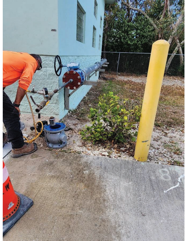
Figure 16 and 17. Pressure testing of force main piping for the VPS job at Vacuum Station D
