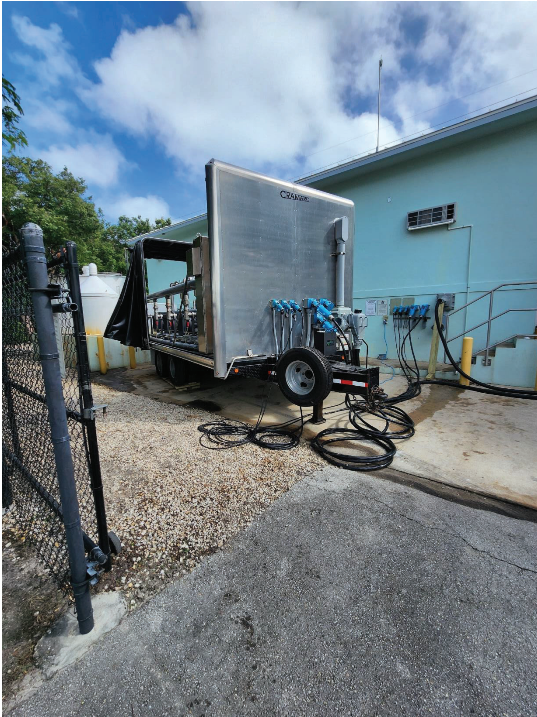
Figure 1. Emergency Vacuum Trailer Connections for VPS Project.
