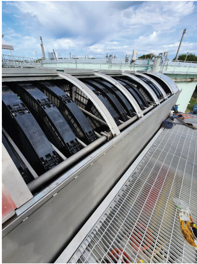
Figure 7. Interior Disk Filters.
