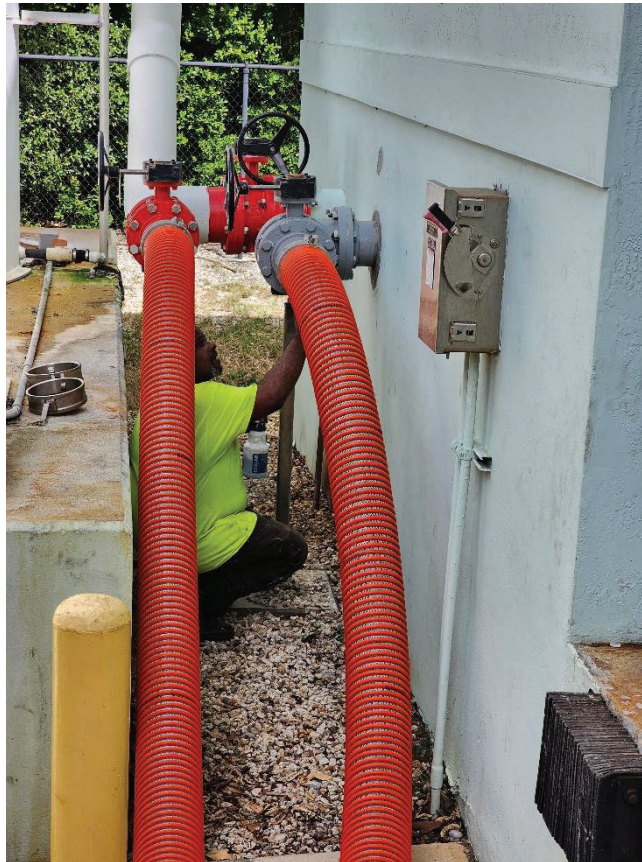
Figure 2 and 3. Emergency Vacuum Trailer Connections for VPS Project.
