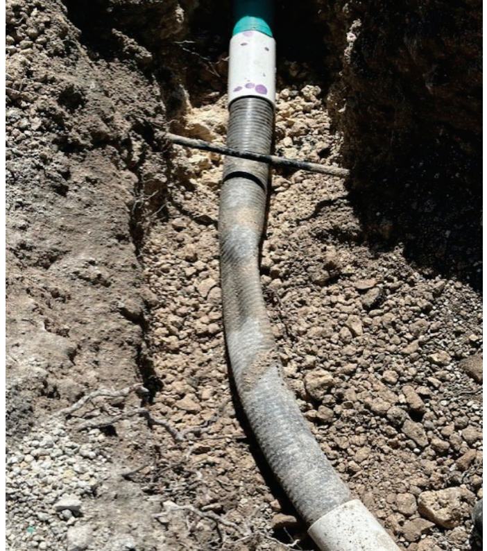
216 Buttonwood Lane: Field techs addressed a 3" collapse vacuum line with the help of a high level alarm from the FloVac monitoring system.
