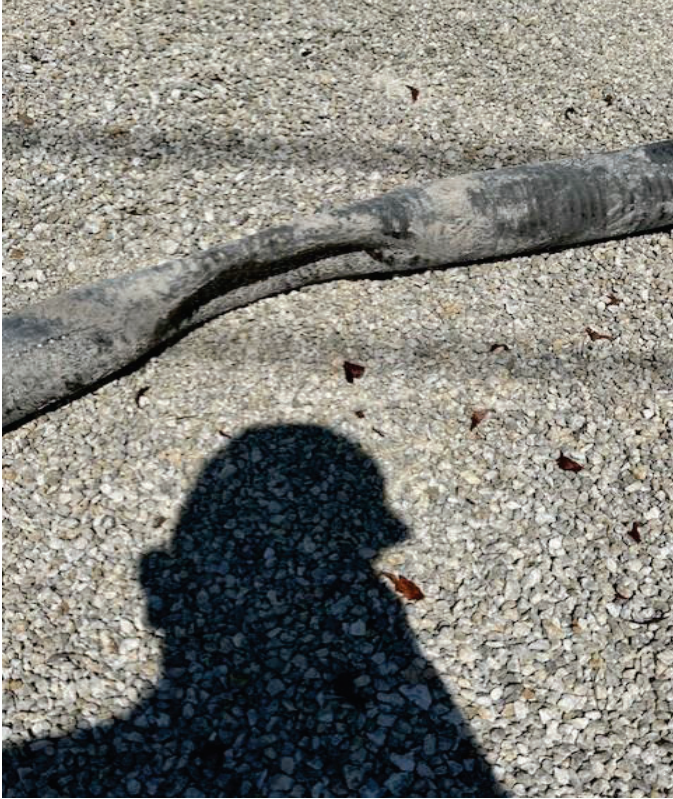
216 Buttonwood Lane: Field techs addressed a 3" collapse vacuum line with the help of a high level alarm from the FloVac monitoring system.
